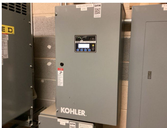
24 - AUTOMATIC TRANSFER SWITCH
