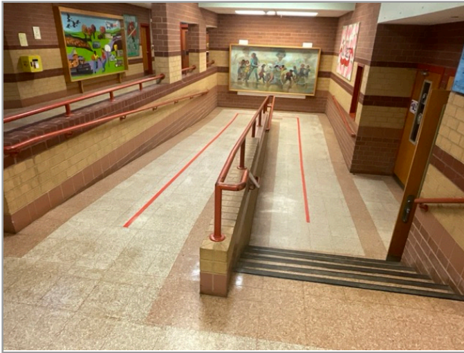
ACCESSIBLE INTERIOR RAMP
